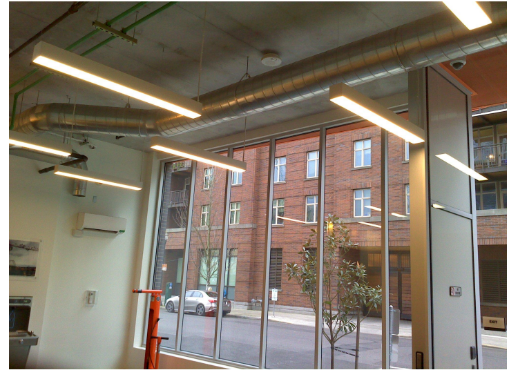
G.L. - Bike Window Type - Curtain Wall FLIR Picture: Data Collection Day #1
